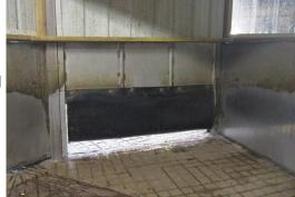
Vertical slide gates constructed from flexible curtain made from conveyor belting will not injure the swine if it is accidentally closed on them. Note how the framework that slides in the track is bolted above the curtain.
